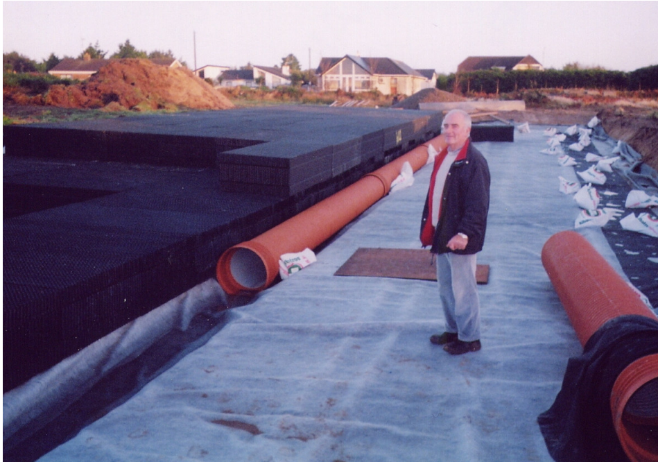
Construction of the tank
