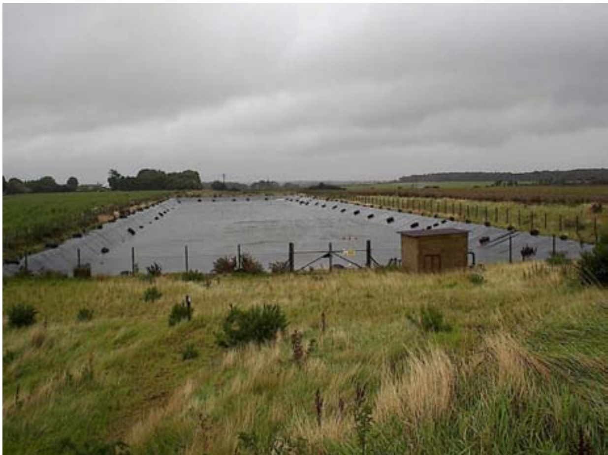
Photo 4: Completed 31,800m 3 reservoir
