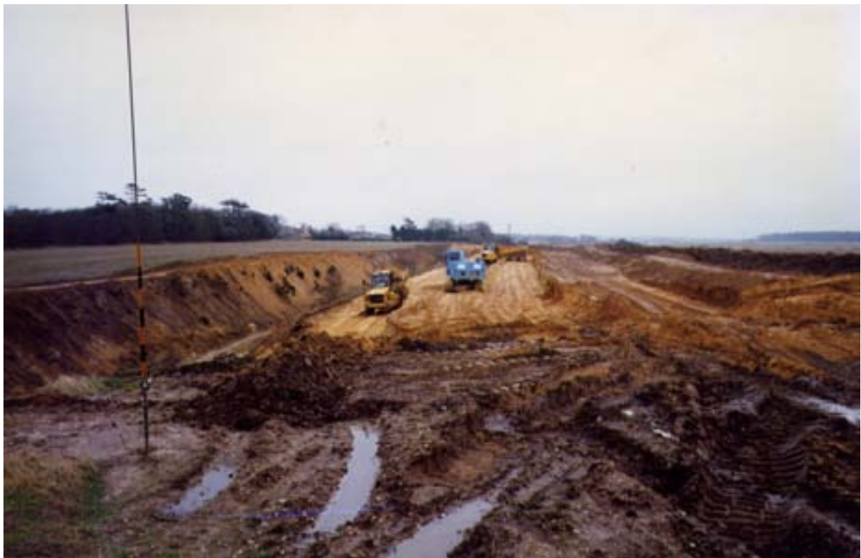
Photo 2: Excavation of cutting and infilling at ends
